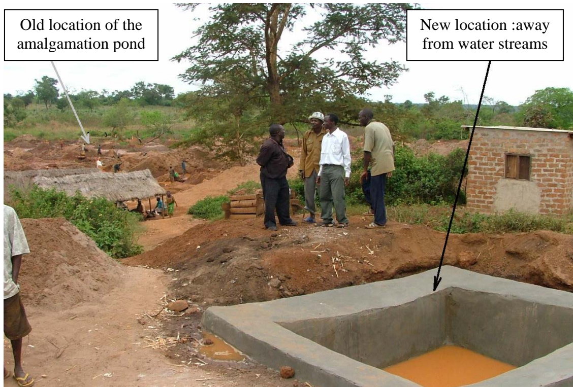
Figure 6: Relocation of washing pond away from the river channel
